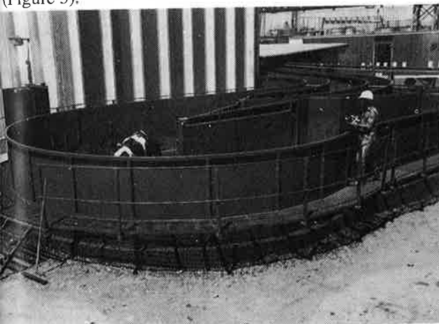
Figure 5. Round forcing pens with solid sides are efficient for moving all species.
