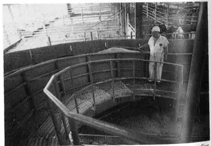
Figure 3. A curved race with a walkway which runs alongside the inner radius is more efficient than a straight race. All races should have solid fences.
