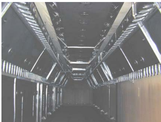
Fig. 1: Newly designed ripening chamber with vertical and horizontal inlet airflow
